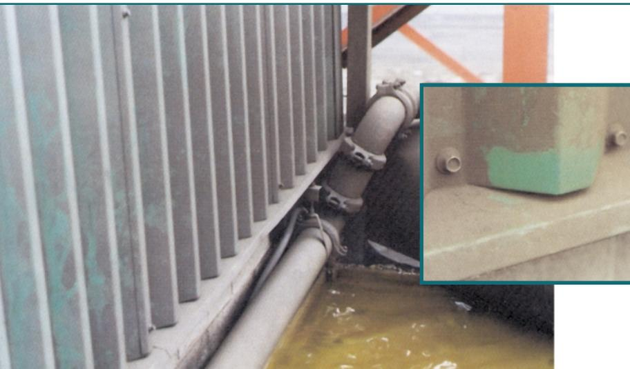
**Figure 1:** Mine water cooling tower. West exposure above the tanks. Insert: A quick cleaning showed that the drip edge was in excellent condition. Eleven years exposure in Northern Ontario.
