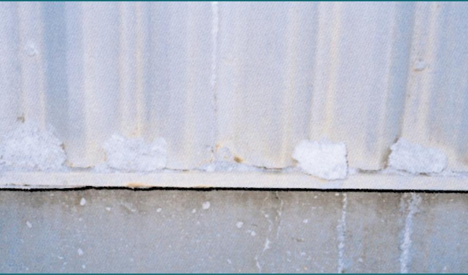
**Figure 4:** Pulp & paper plant, recovery boiler building. Ground level west exposure below exhaust duct showing contaminate build-up and minor edge creep on the cladding. Eleven years exposure in Northern Ontario.
