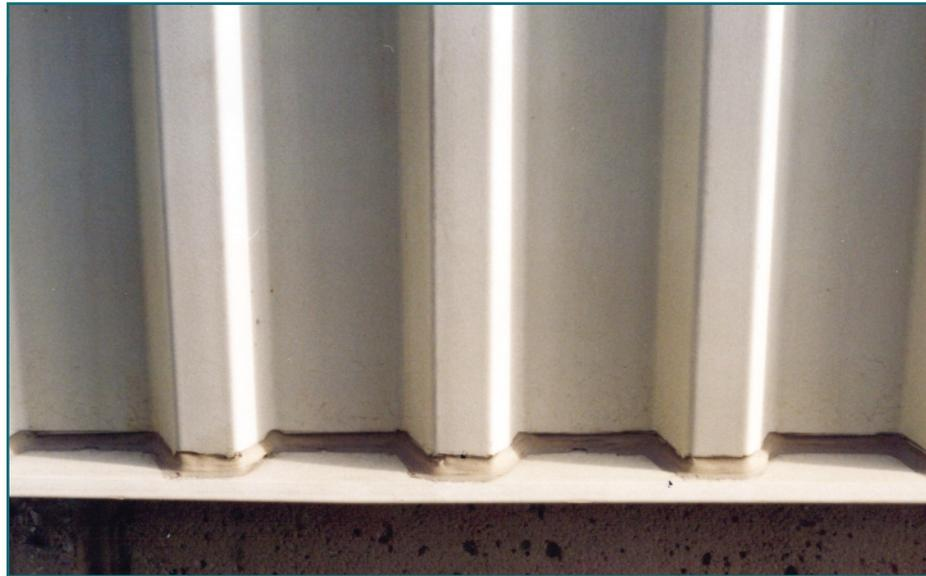
**Figure 9:** Example of effective edge sealing with caulking on an exterior wall.
