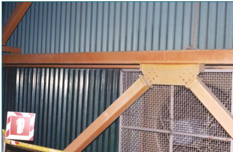
**Figure 3:** Mine refinery building interior. The Barrier Series cladding is above the exhaust fan. Eleven years of exposure in Northern Ontario.
