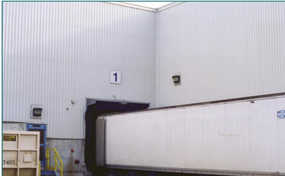
**Figure 6:** Kraft fine paper plant, paper finishing building. Comparison of new and old nine-year cladding. The newer cladding is on the right. Location in Northern Quebec.
